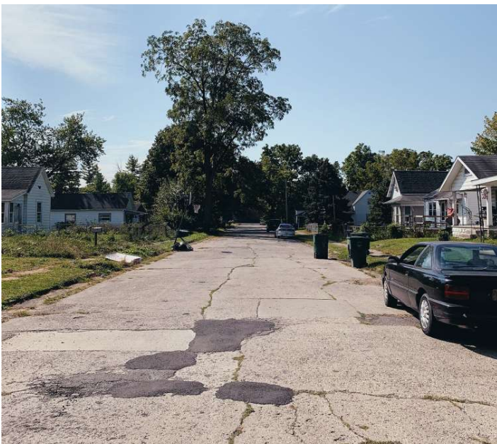
Figure 43: Side Road in Southside Neighborhood. Source: Carter Solivan
