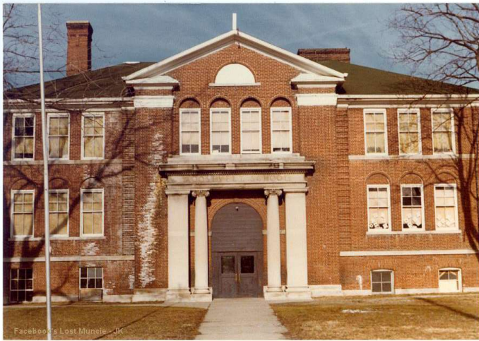
Figure 20: Roosevelt Elementary School. Source: https://www.facebook.com/photo
