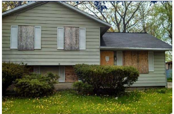
Figure 37: Example of a Poor House Condition source: https://www.usfa.fema.gov/current_events/041718.html
