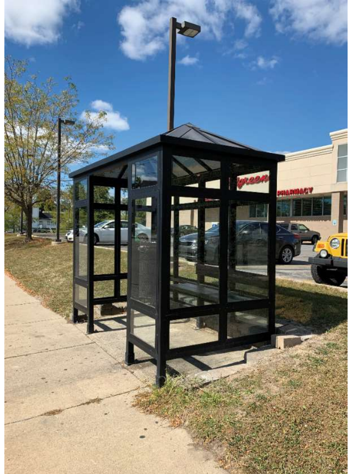
Figure 39: Bus Stop on Madison and Memorial. Source: Alex Pope
