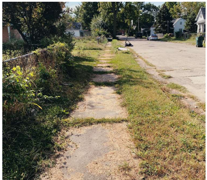
Figure 42: Overgrown Sidewalk. Source: Erick Portillo
