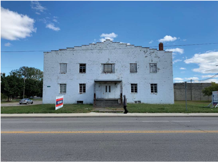
Figure 32: Abandoned Building Currently. Source: Carter Solivan
