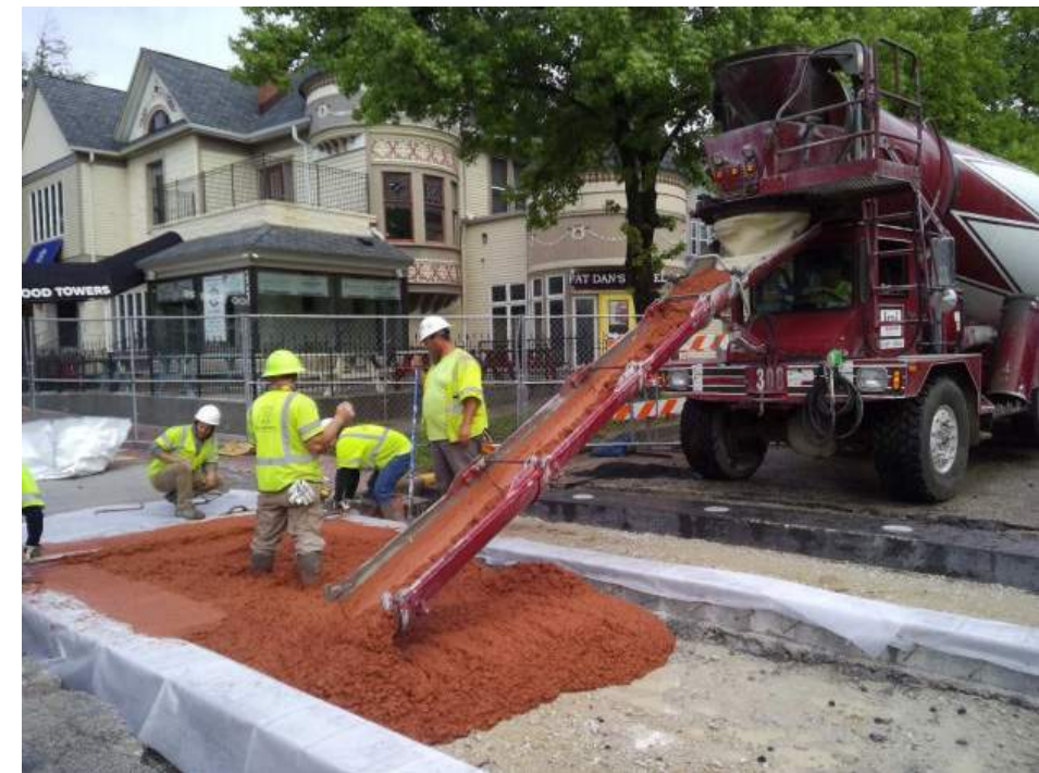
Figure 67: Kirkland Crosswalk Construction
