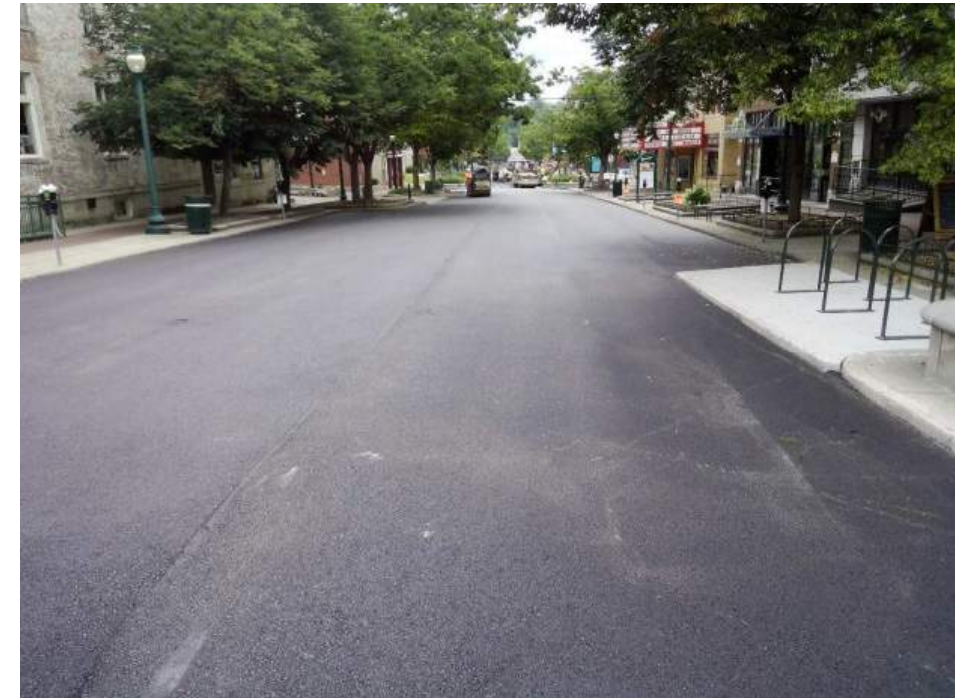
Figure 66: Kirkland Street Reconstruction
